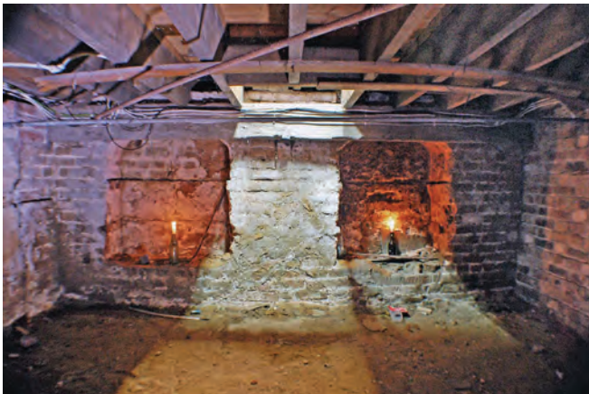
Storage bays and the trap down from the shop, formerly the White Lion, above
